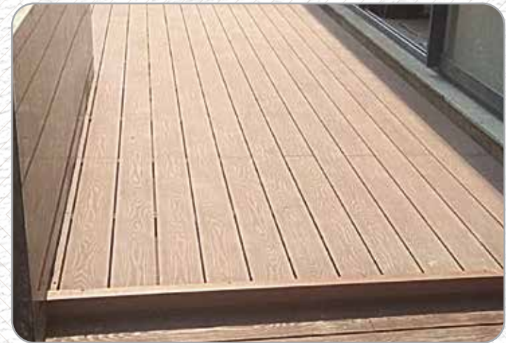
WPC USED IN WOODEN DECK AREA
