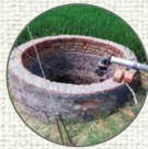
Common wells connected to a common sump
