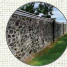
Designer compound wall facing ECR
